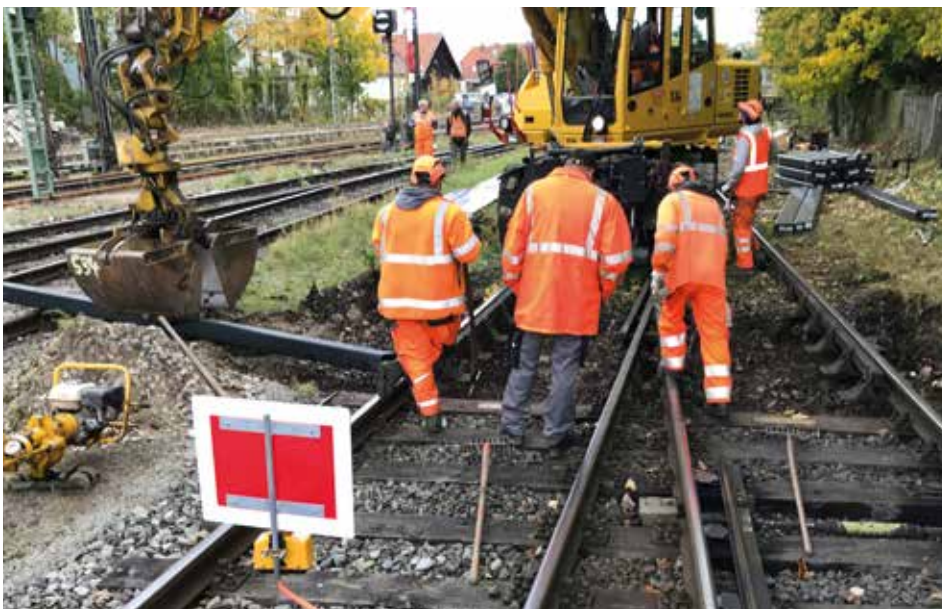
Figure 3 Pose des traverses composites STRAILWAY .
