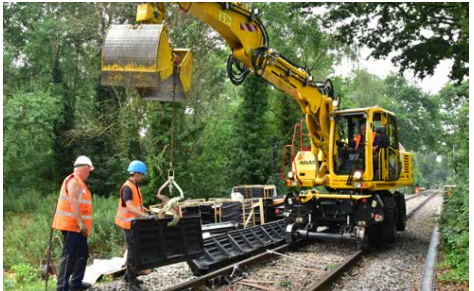
Montage STRAILastic_mSW
