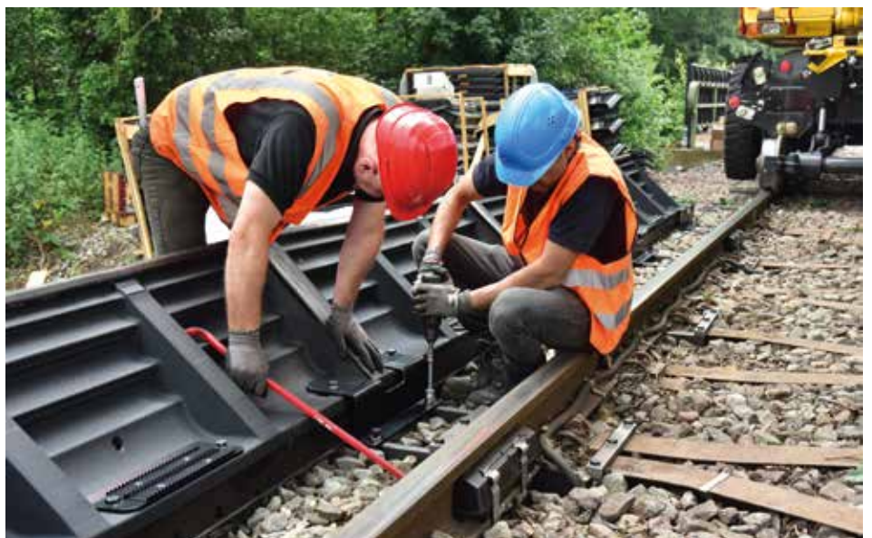
Montage STRAILastic_mSW
