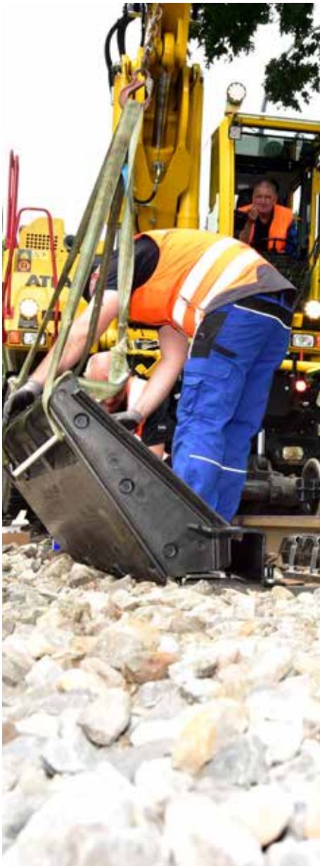
Montage STRAILastic_mSW
