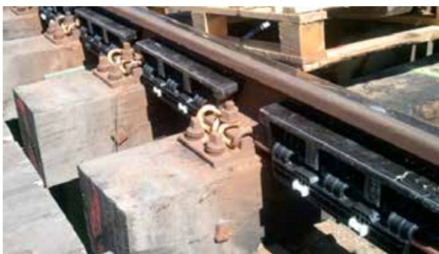
Éléments STRAILastic_A installés
