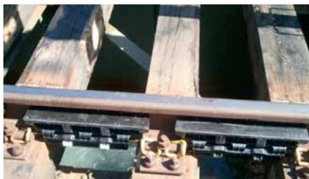
Éléments STRAILastic_A installés
