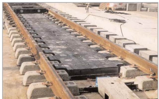
Covering for the steel sub-structure
