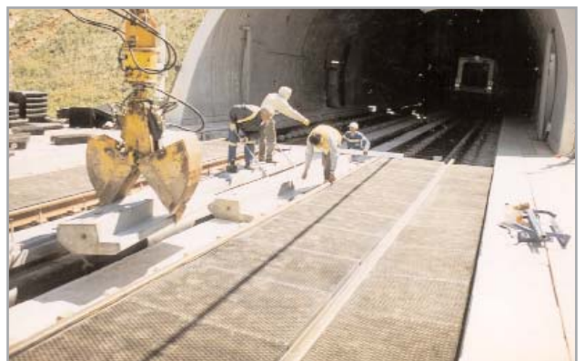
Laying the concrete kerbstones
