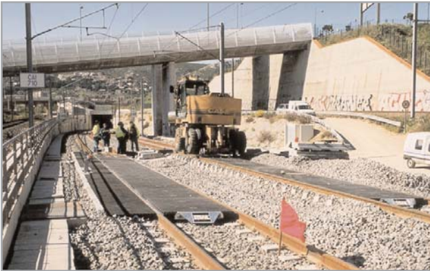
View in the direction of the tunnel
