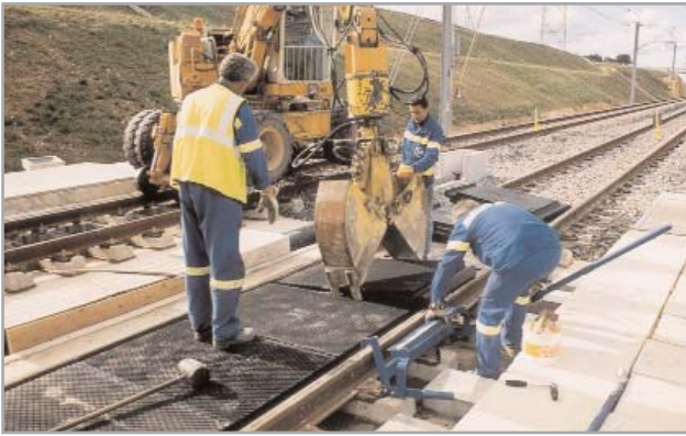
Assembling the inner panels
