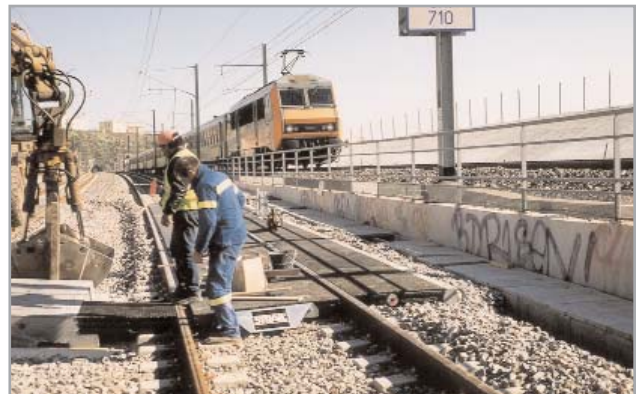
Fitting the outer panels in the area between the tracks
