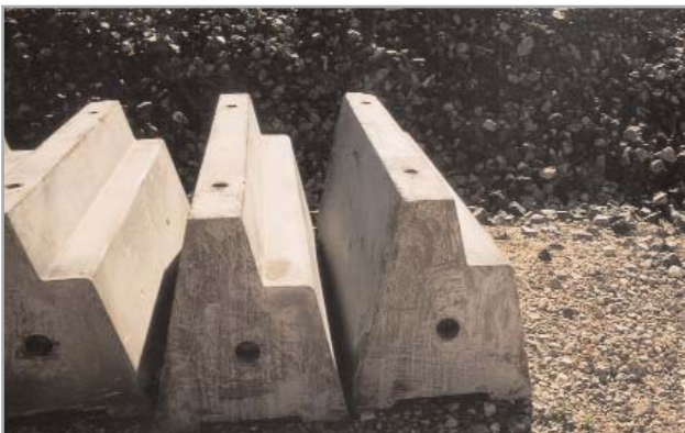
Concrete kerbstones for outer panels
