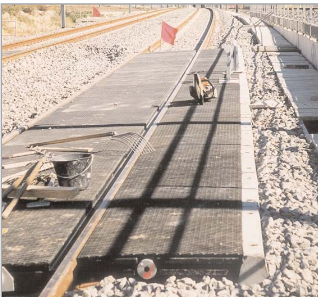
Concrete kerbstones for outer panels
