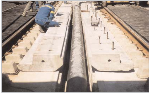
Bridging the drainage pipeline out of the tunnel
