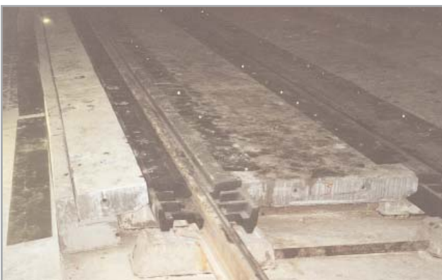
STRAILprofil combined with concrete panels in the inside of the tunnel
