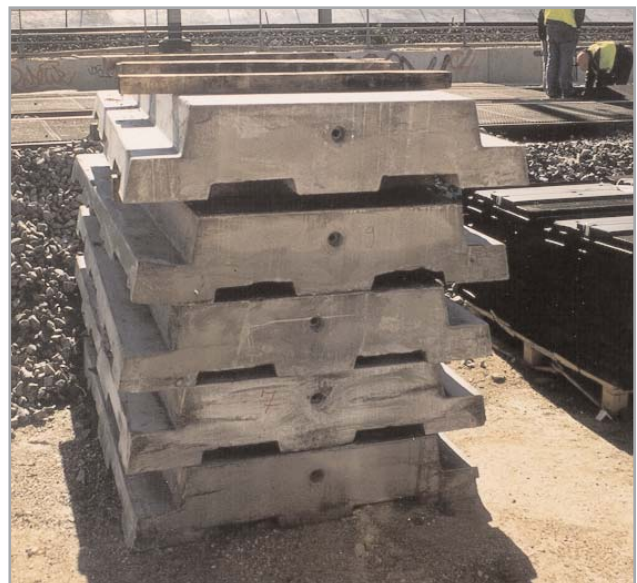
Concrete kerbstones for the area between the tracks
