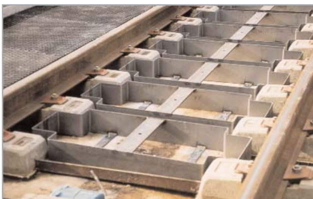
Steel sub-structure in the inner area
