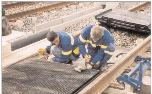
Fixing the panels with bolts and tie rods
